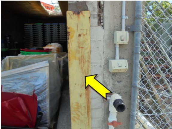
Photo 1. Exterior, east elevation, metal framework - suspected lead-containing yellow upper paint system.
